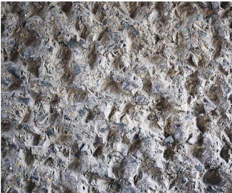
△ Pick-hammered concrete surface ▷ Lauderdale Tower from Lauderdale Place
