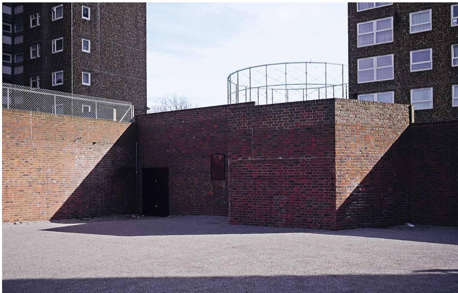
Ledbury Estate ◁ Sarnesfield House, from Old Kent Road ▷ Sarnesfield House, Skenfrith House and communal area
