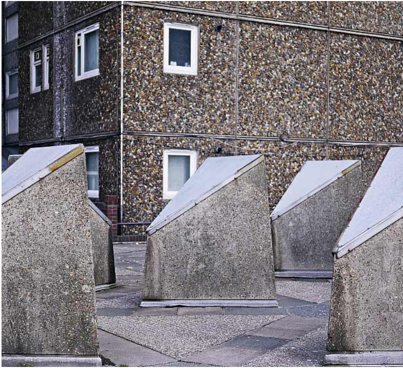
Sarnesfield House and covered vents
