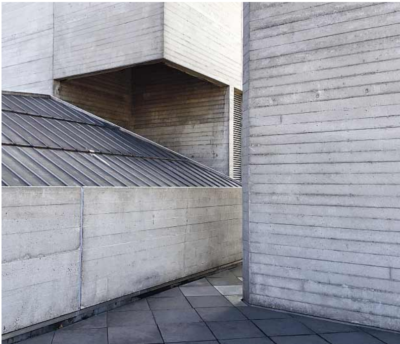
Board-formed concrete
